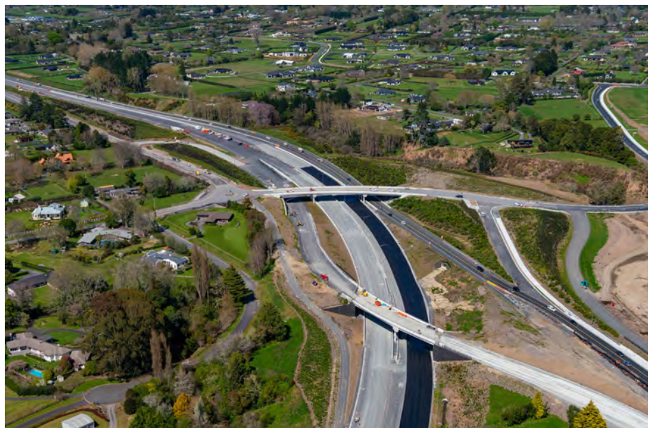
The Hamilton section of the Waikato Expressway joins the exiting SH1 at Tamahere where a lot of work has been done to keep local people connected, with ramps on and off the expressway and roads extended.
